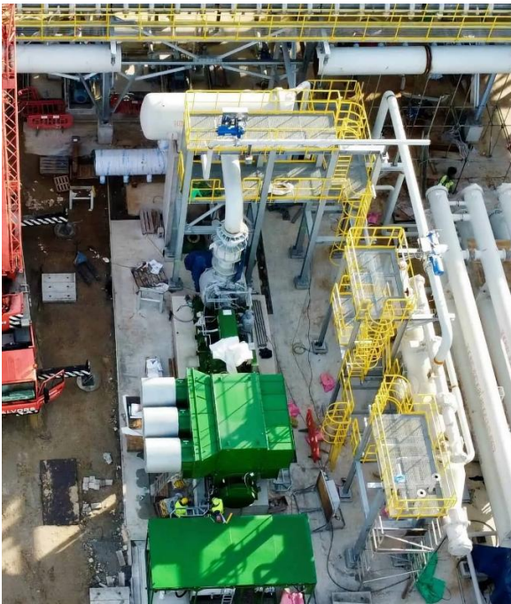
Figure 5: United Downs Geothermal Plant Construction Site
