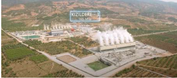
Figure 3: Kızıldere-III GPP units (by Zorlu Enerji)
