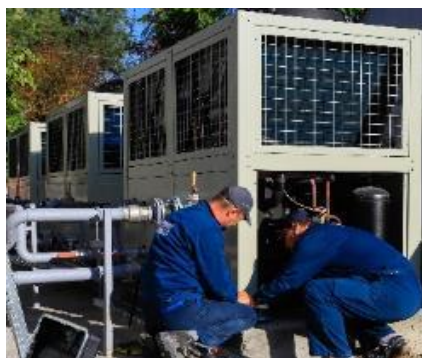
Figure 7: The installation of the innovative recovery tank Smart Campus University Oradea I
