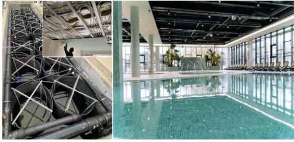
Figure 9: The geothermal wastewater recovery tank (left) and the inside pool of the hotel (right)
