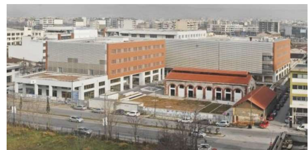
Figure 2: The new building of Central Macedonia Regional Authority (Thessaloniki, N. Greece)
