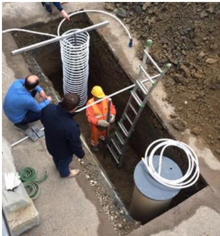
Figure 4: Installation of the two Spirals in the test site.
