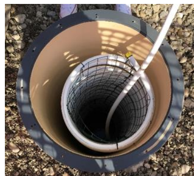
Figure 2: Helical heat exchanger (Spiral) in the casing.
