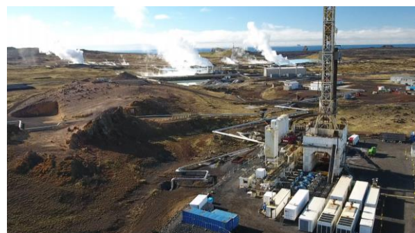
IDDP-2 DEEPEGS demonstrator well at Reykjanes.
