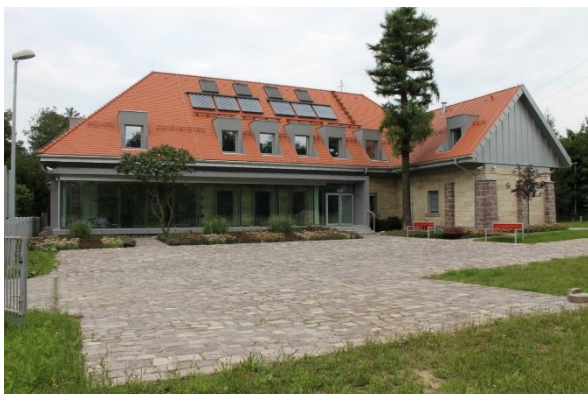
Figure 1: The building of the AGH-UST Educational and Research Laboratory of Renewable Energy Sources and Energy Saving in Miękinia.
