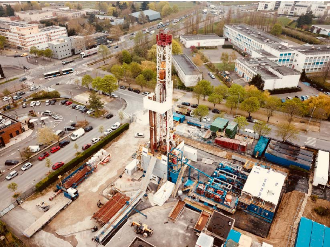
Figure 6: Bonneuil-sur-Marne drill site aerial view (courtesy of SMP)
