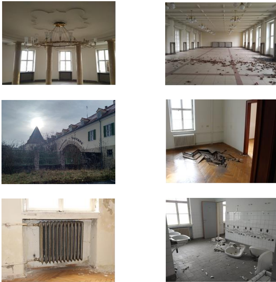
Figure 3: Pictures of the interior of the buildings and the outside area. The central staff building with the main entrance and the round tower is well-preserved. The upper two pictures show the dining hall and the main meeting room in the round tower. In some pictures, the poor condition of the buildings – partially due to damage by water - even after only four years of abandonment and signs of vandalism can be seen.
