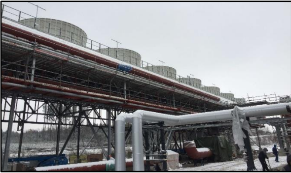
Figure 5: Holzkirchen geothermal plant
