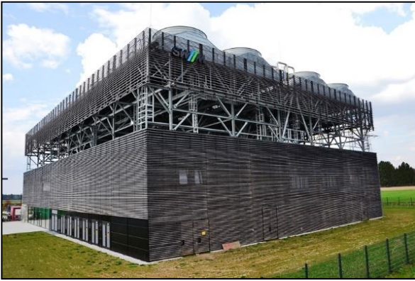
Figure 1: Sauerlach geothermal plant
