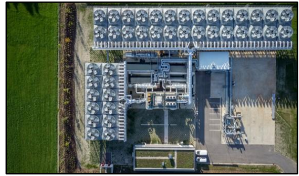
Figure 3: Dürnhaar geothermal plant
