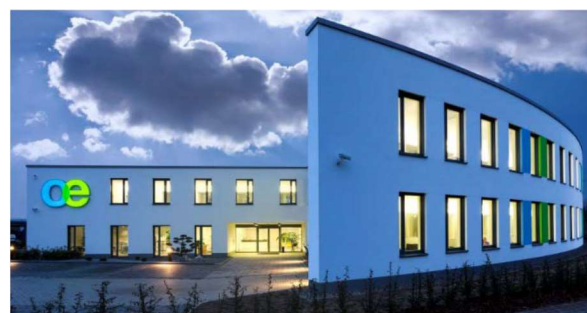
Figure 7: Facilities of oeding print GmbH in Braunschweig-Rautheim (photo oeding print).
