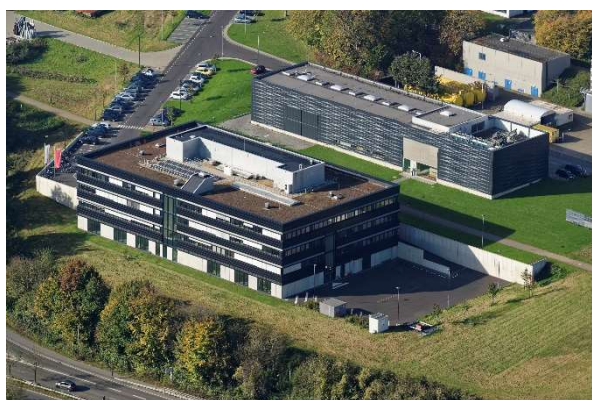
Figure 4: E.ON Energy Research Center at RWTH Aachen; the 40 BHE are grouped in 3 fields around the building (photo E.ON-ERC).
