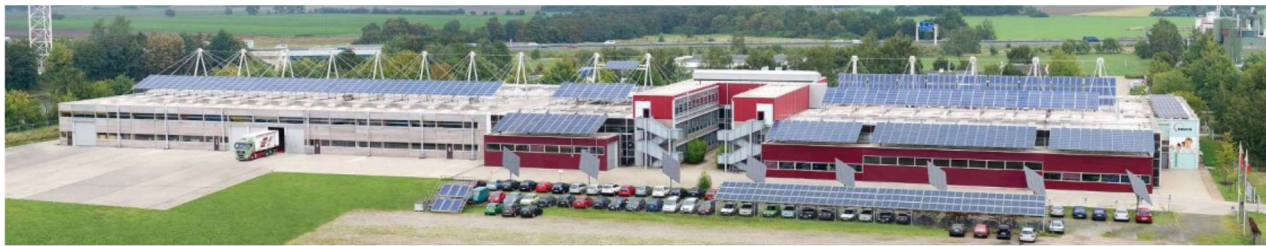
Figure 8: Zero-emission factory of SOLVIS GmbH in Braunschweig, with solar energy and water storage (photo SOLVIS).
