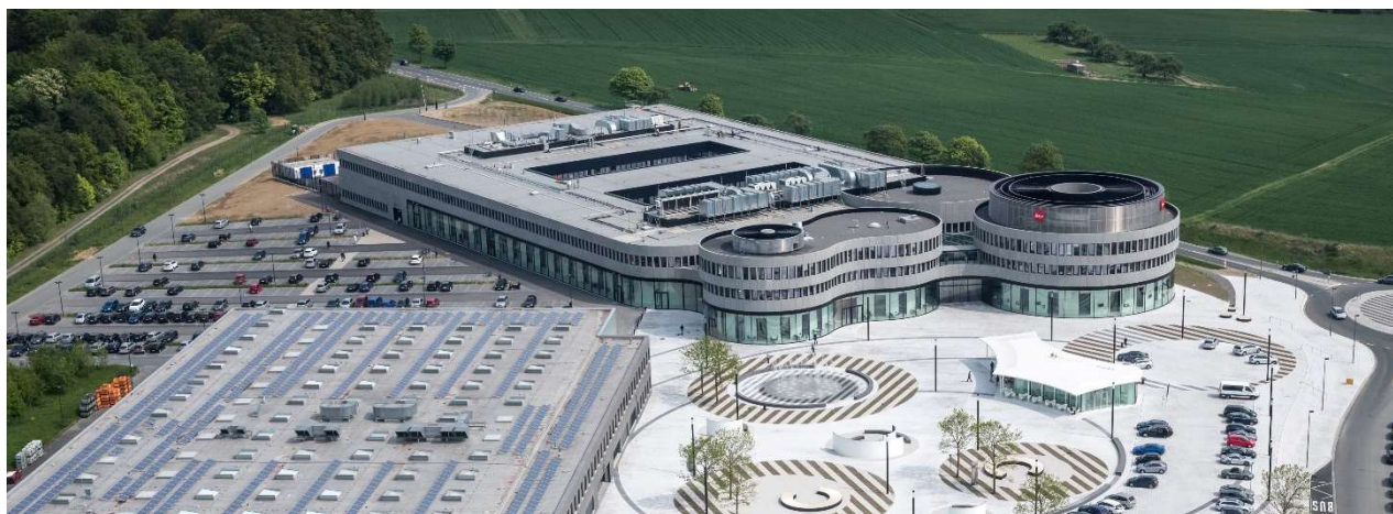
Figure 6: The Leica Camera AG offices and factory in Wetzlar, shortly after inauguration in 2014; the two BHE fields are located under the parking to the left (photo Leica Camera AG).
