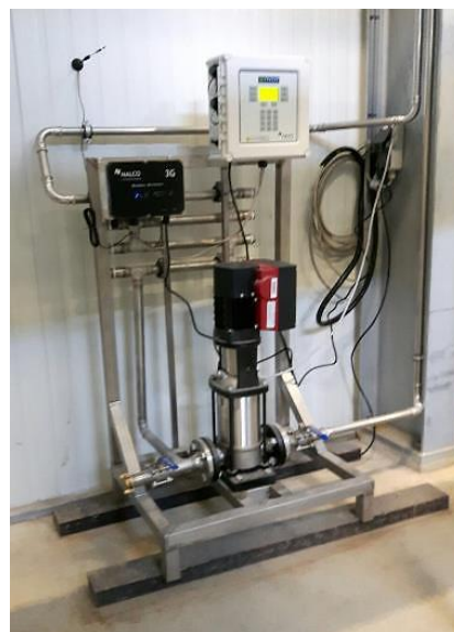
Figure 6: Corrosion monitoring device, 3DTRASAR for Geothermal.
